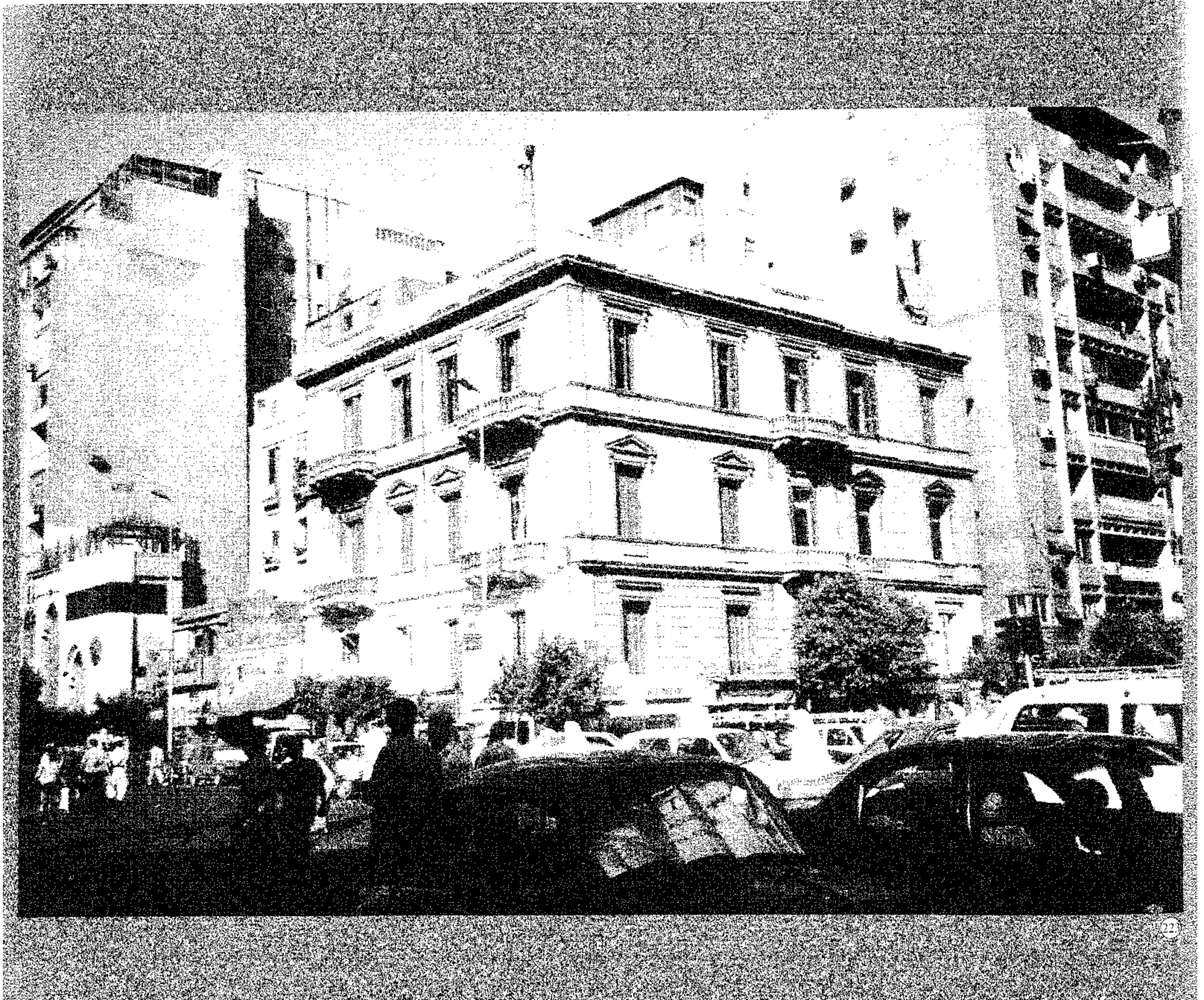
10/11 Suliman El-Halabi St. Corner of Orabi St. & Suliman El-Halabi St. Built : beginning of 20 th Century Area : 405 m 2 No. of stories : 4 Style : Classic
